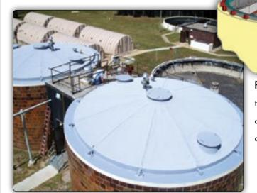
**Fixed digester covers** are anchored to the top of the tank walls and are typically used on primary digester tanks operating with constant sludge levels.
