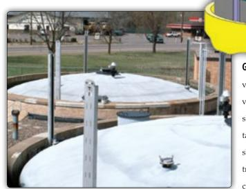
**Gasholder covers** move up and down with varying sludge level and with changes in gas volume stored. They are used for gas and sludge storage, often on secondary digester tanks. OTI's innovative, maintenance-free slide/guides, for even and balanced cover travel, are designed for all specific operating conditions.
